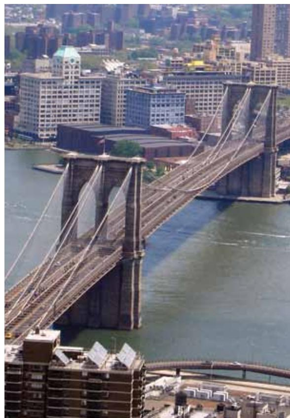
**The Brooklyn Bridge, opened 1883, is perhaps the most recognized natural cement structure in the world. Natural cement concrete, mortar and grout were used in its construction.**
