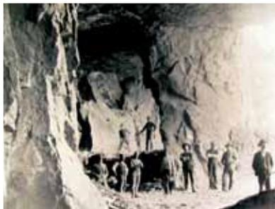
**Natural Cement Mine, circa 1890. Room and pillar mining techniques were most commonly used in natural cement rock mining.**
